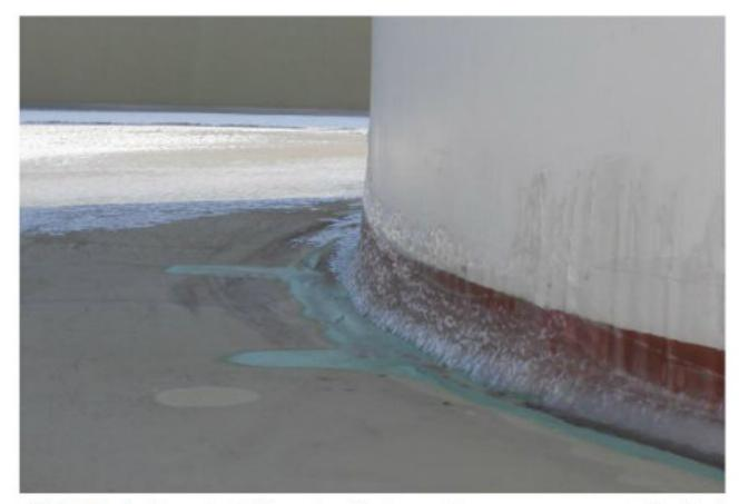
ABOVE At a tank farm in Alaska polyurea over geotextile had served well as secondary containment for 17 years, but eventually the harsh environment took a toll on the liners. "With the wind uplift and the salt water environment, the seams in the liners were starting to tear and delaminate," says Morrow.
